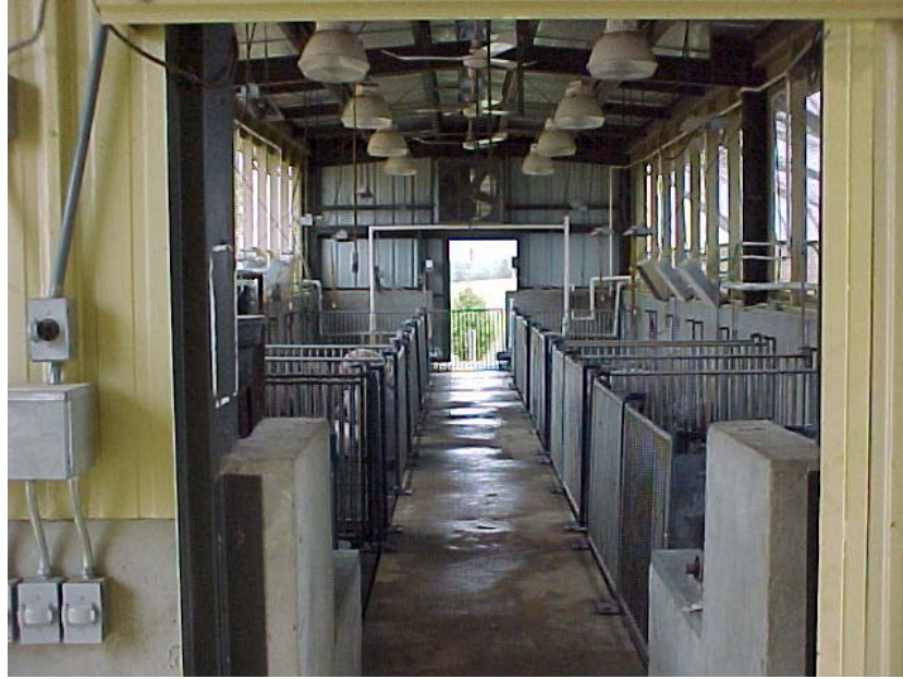
Figure 3.3. Inside view of barn
