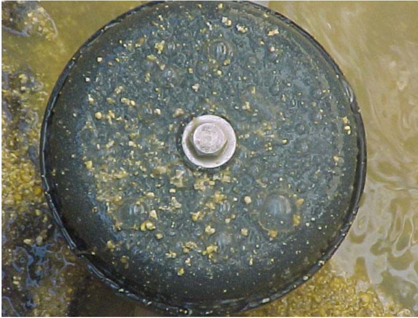
Figure 3.8. Ceramic diffuser used in the aeration system
